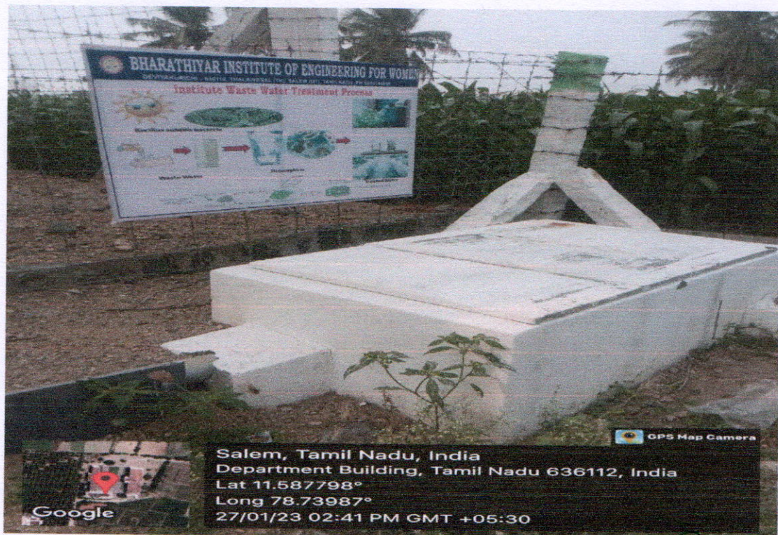
Microbial waste water treatment plant located in the campus
